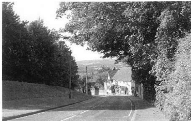
Linton Hill in 2007, showing the road running through the cutting created when the turnpike road was regraded in the 1830s.
