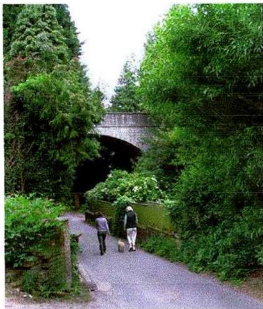
The Loose Viaduct spanning the Loose Stream and Salts Lane.
